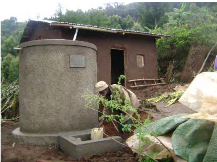
Photos: Kaburabuza at his house before renovation and after renovation with the tank constructed by KDWSP
